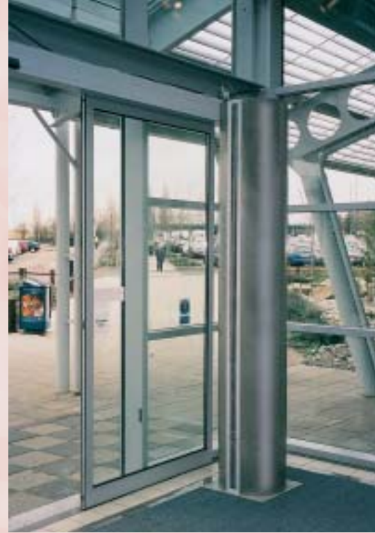
One of a pair of 2800 x 500mm vertical CDC Door Curtains installed at the entrance to a motorway services development, finished in brushed stainless steel
